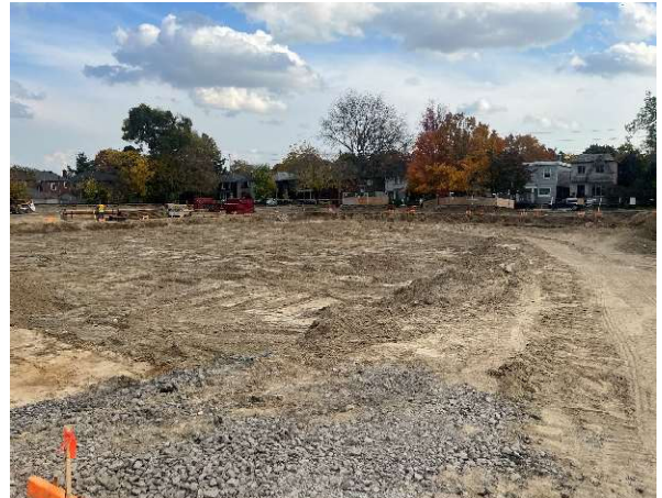
Exterior photo showing the excavation progress of the future 3 storey addition.
