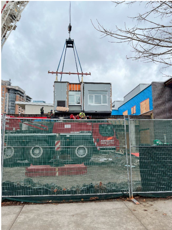
Confirmation of drop in and tie in of second modular unit.
