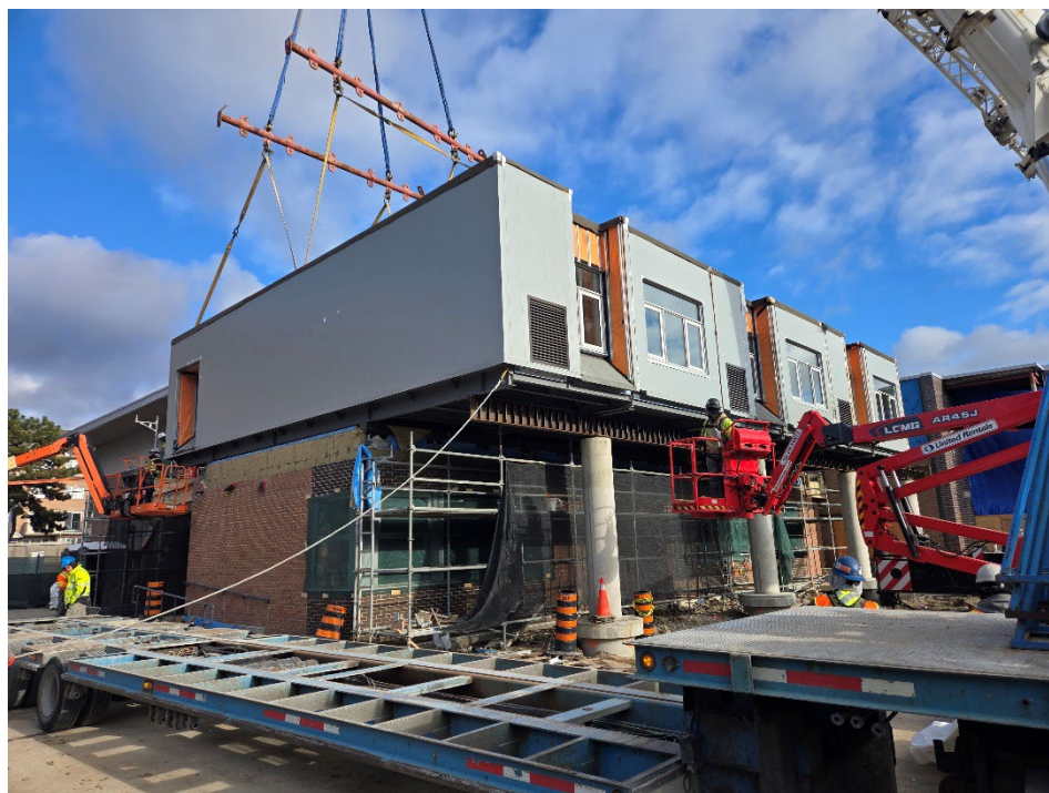
All six modular units installed in place.
