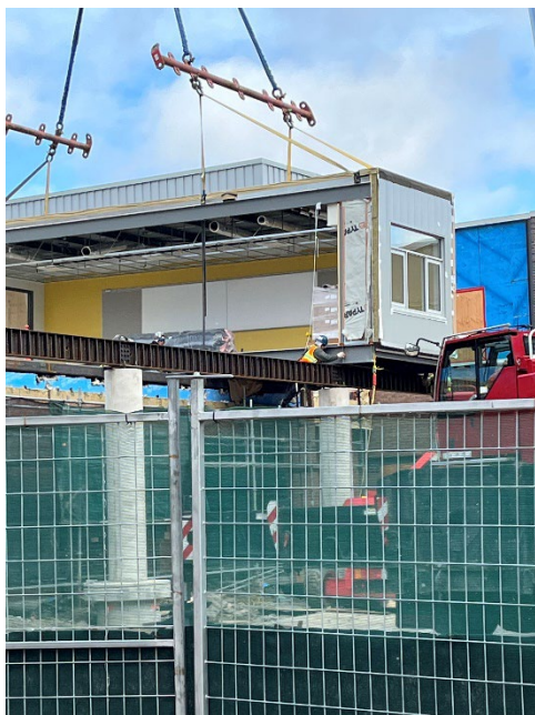
Drop in place and tie in of first modular unit
