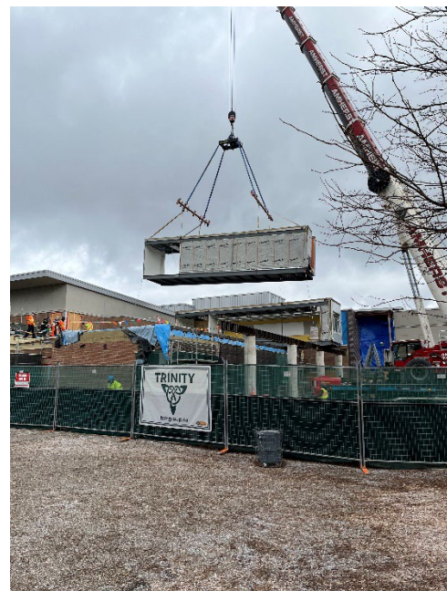
Lifting of second modular unit
