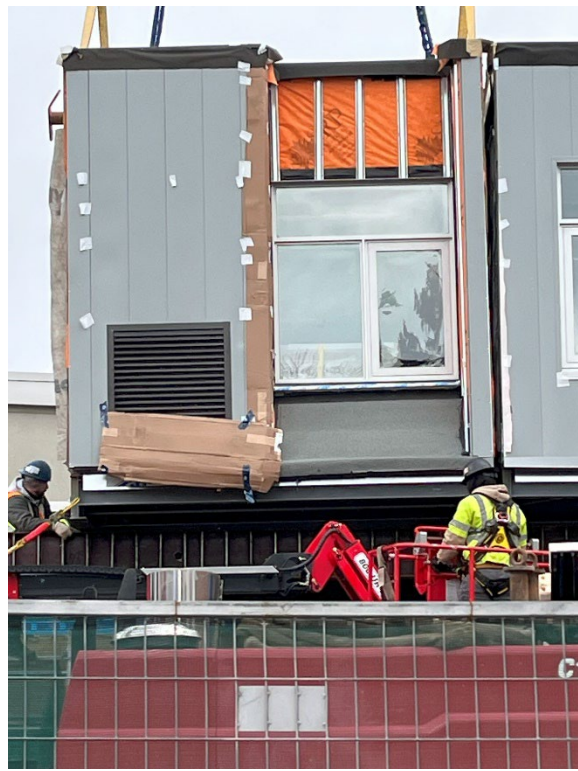
Confirmation of drop in and tie in of second modular unit.
