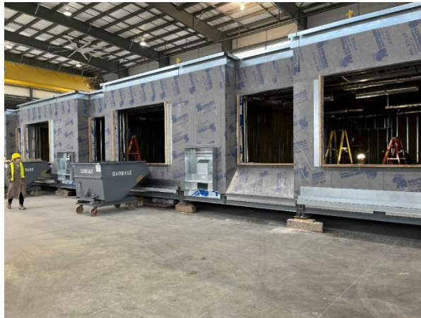
3 classrooms being constructed offsite by the Modular Manufacturer
