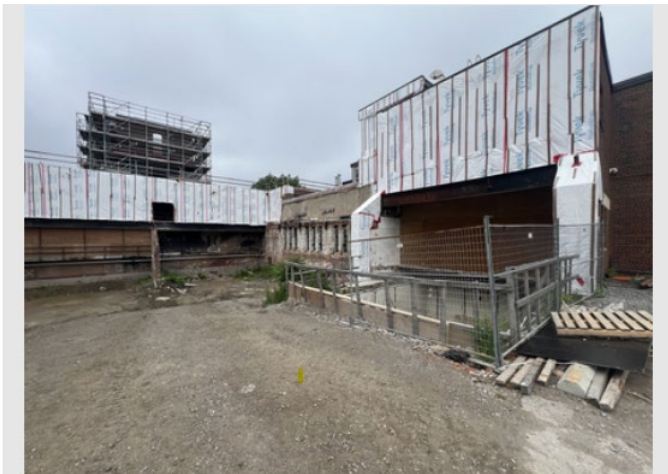
Additional Shoring, scaffolding, and bracing:
