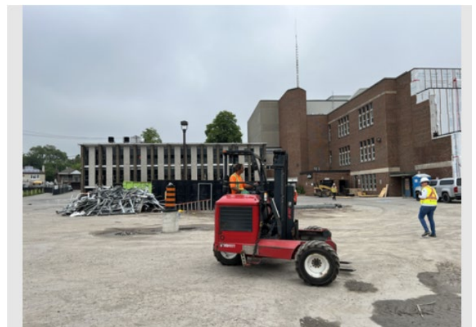
Beginning of demolition of the Annex:
