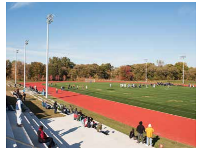
TOP: Perched at the corner of the fourth floor, the library is an expressive feature along the south elevation, recognizable from a distance as a beacon for the school. BOTTOM: Exterior facilities include a field house, an eight-lane synthetic track circuit and multiple artificial turf play fields capable of hosting the highest calibre athletic event.
